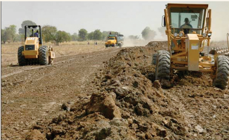
Road construction in Nairobi, Kenya by Chinese contractors
